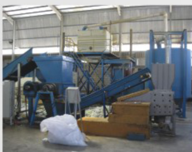
Complete Image of Re-Bounding Foam Making System
